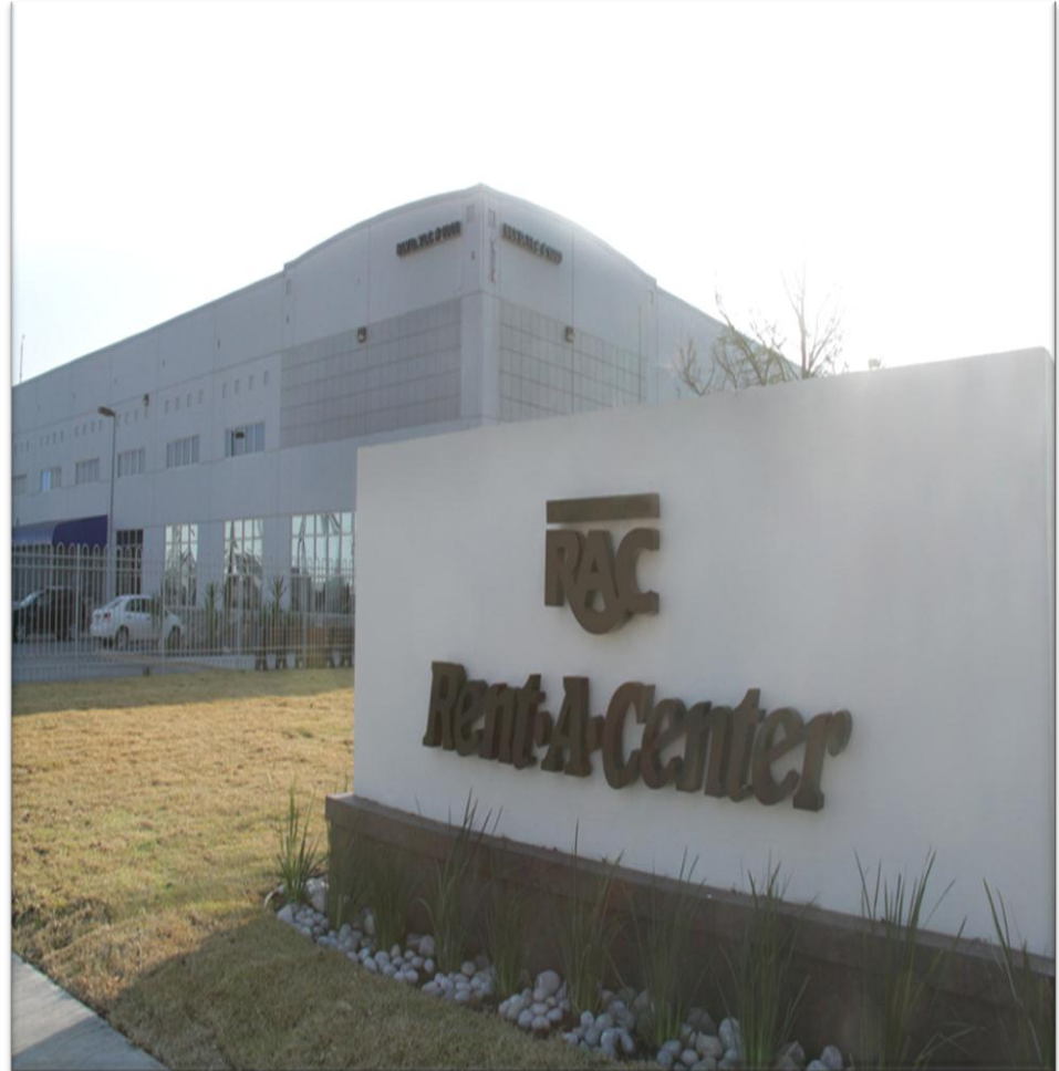
Field Support Center Monterrey, MX
